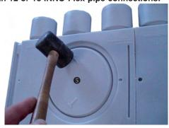
Flip the lid 5 with a medium-strong hammer hit each on the bottom and the top of the connected body, as described under 4.
