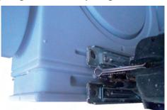
Disconnect the inspection cover on the edge of **1** with a jigsaw cleanly. The sawed-off part is the revision cover dar.
