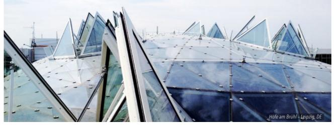
With its low profile height, its large sash dimensions and its specific sealing technique, the WING 105 DI skylight is the perfect solution for almost any application with an inclination down to 2° from horizontal.
