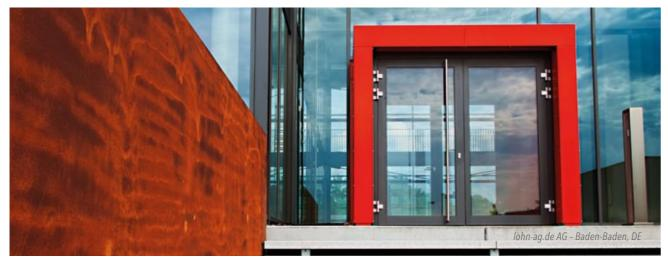
FRAME<sup>+</sup> 75 DI fulfils all the requirements for a high quality entrance door. Special profile contours enable simple installation. The series is characterised by short production times and efficient manufacturing. Smooth rebate geometries enable fast installation of all types of hardware in the rebate. Large internal chambers within the profiles provide acceptance of all fittings, such as electrical door release mechanisms.
